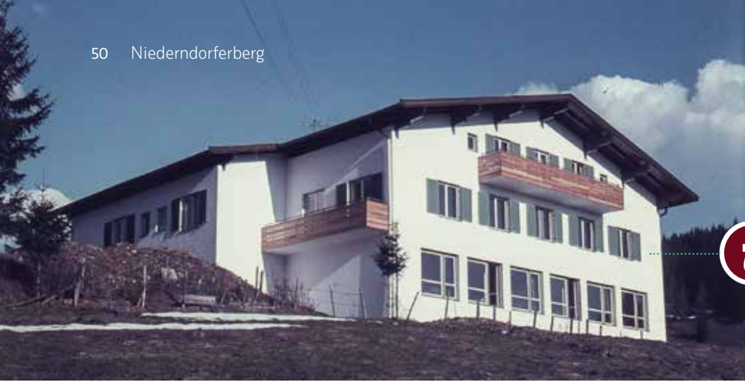
The 'new' school which was built in 1965.
