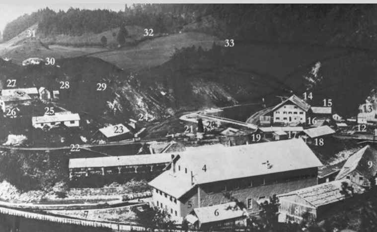
Cement was being fired in the community of Schwöich as far back as 1840.
